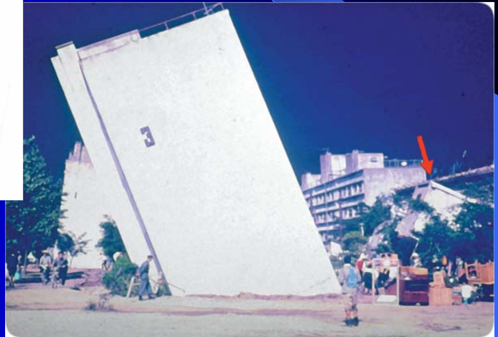
1964 Niigata, Japan Earthquake
