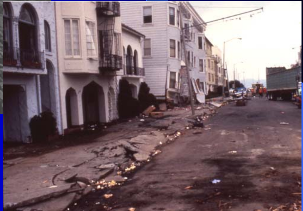
Marina District, San Francisco, 1989 Loma Prieta Earthquake
