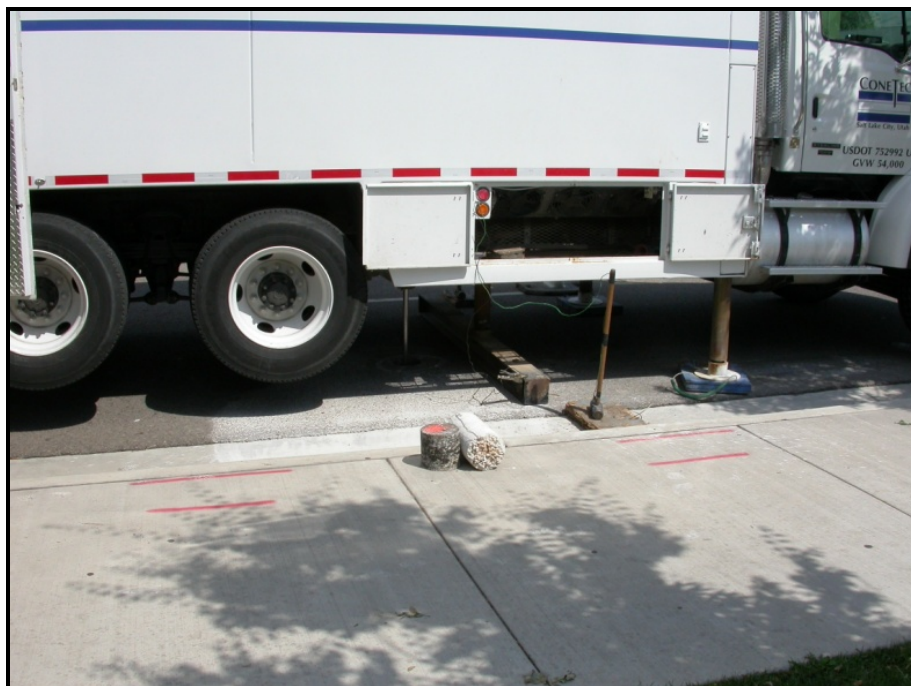
Figure 47 – (CP-7) 20-Ton CPT Rig advancing the cone
