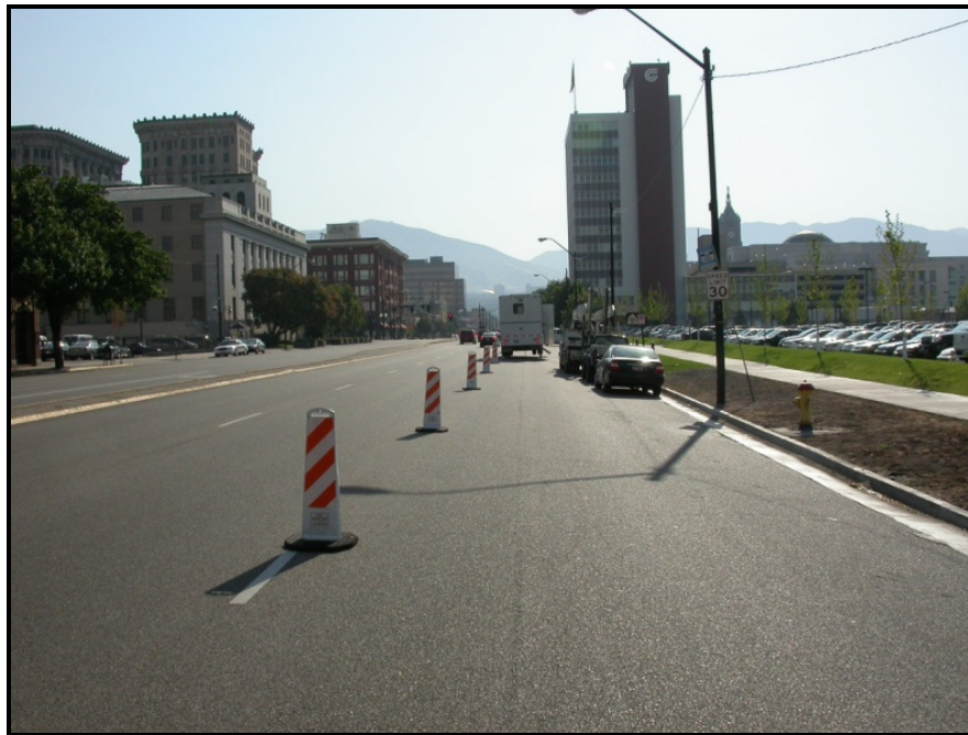
Figure 45 - (CP-4) Lane closure on 400 S, Wells Fargo Building in Background
