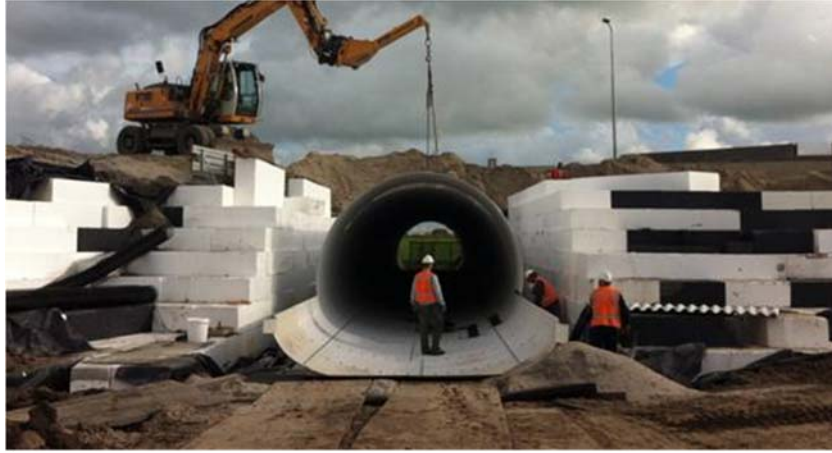
Fig. 27. Construction of corrugated steel tunnel in EPS fill
