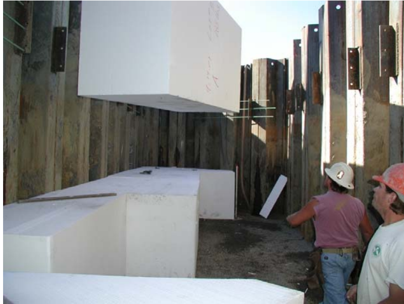
Fig. 20. Geofoam placement within the sheet pile cell
