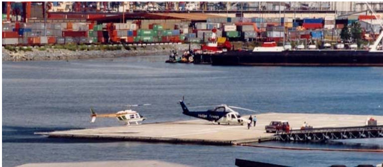
Fig 12. Floating helipad supported by Geofoam blocks in Vancouver, Canada
