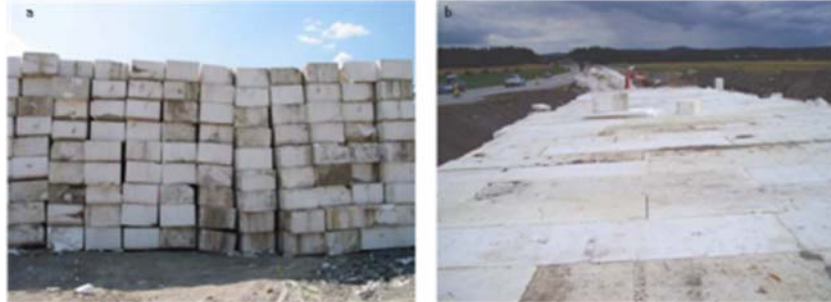
Fig 35. A Stockpile of EPS from Løkkeberg Bridge, b Reuse of EPS blocks from Løkkeberg Bridge (NPRA)
