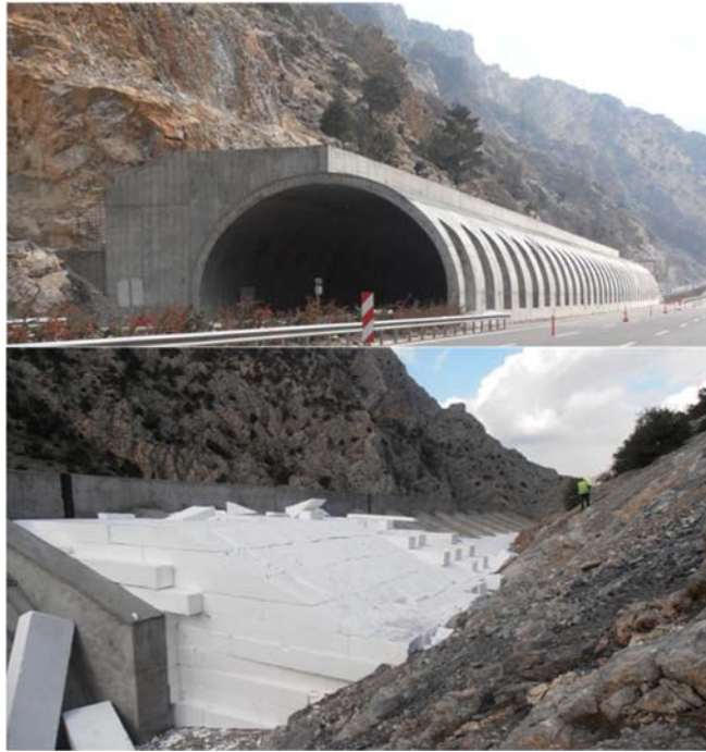
Fig. 23. Geofam blocks applied for energy absorption on rock fall protection tunnel in Turkey (Courtesy of EPSDER, Turkey)
