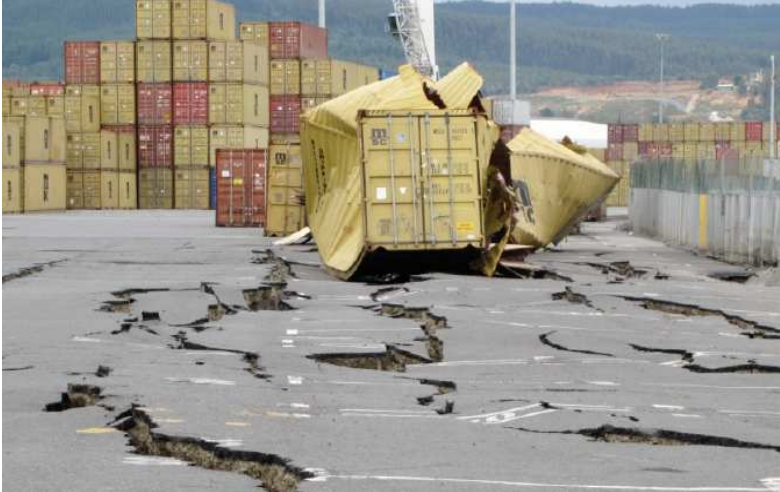
Figure 24: Lateral spreading damage from the 2010 magnitude 8.8 Chile earthquake. (Technical Council on Lifeline Earthquake Engineering - TCLEE)
