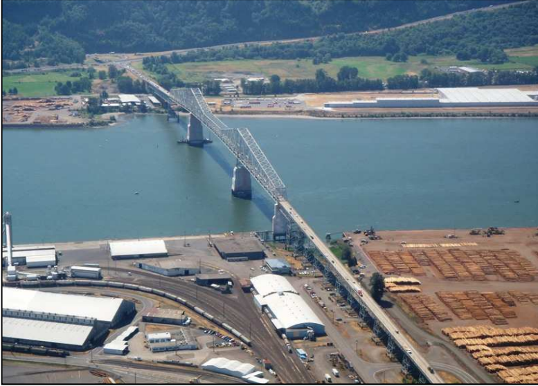
Figure 52: 1930 Lewis and Clark Bridge in the Longview, Washington area crosses the Columbia River (DOGAMI photo)
