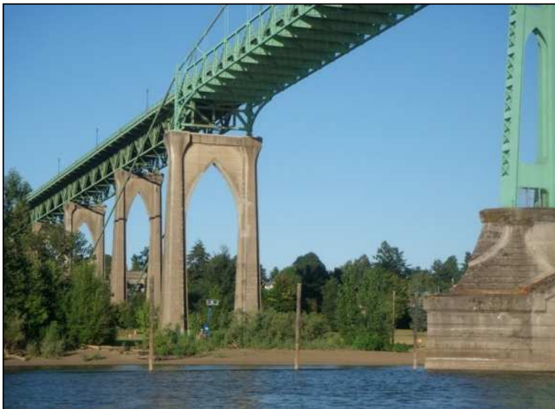
Figure 55: The 1931 St. Johns Bridge crosses the Willamette River in the CEI Hub. The tall columns that are part of the approach are seismically deficient. (DOGAMI photo)
