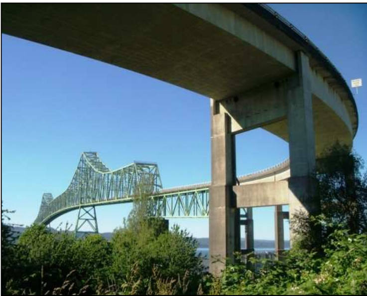
Figure 49: The approach (foreground) to the 1966 Astoria-Megler Bridge that spans the Columbia River has major structural deficiencies according to ODOT Bridge Section. In a major Cascadia earthquake, the exterior (concrete) shear keys on the approaches would likely not withstand lateral displacement of the superstructure (approach deck) (DOGAMI photo)
