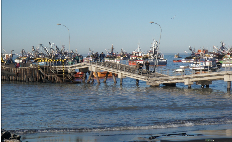
Figure 44: An example of a damaged pier in the 2010 Chile earthquake (Technical Council on Lifeline Earthquake Engineering – TCLEE - 2010)
