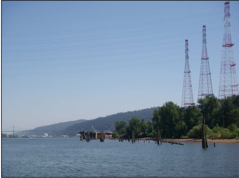
Figure 54: The high voltage electrical transmission crossing showing transmission towers built on a river bank susceptible to lateral spreading (BPA, 2008) (DOGAMI photo)
