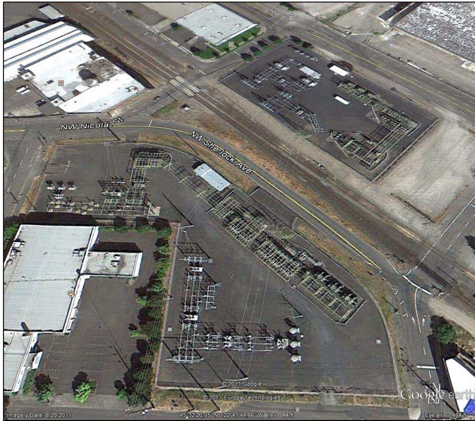
Figure 32: Two large electric substations just south of the CEI Hub on Front Street that are separated by a railroad track (Basemap: Google Earth)
